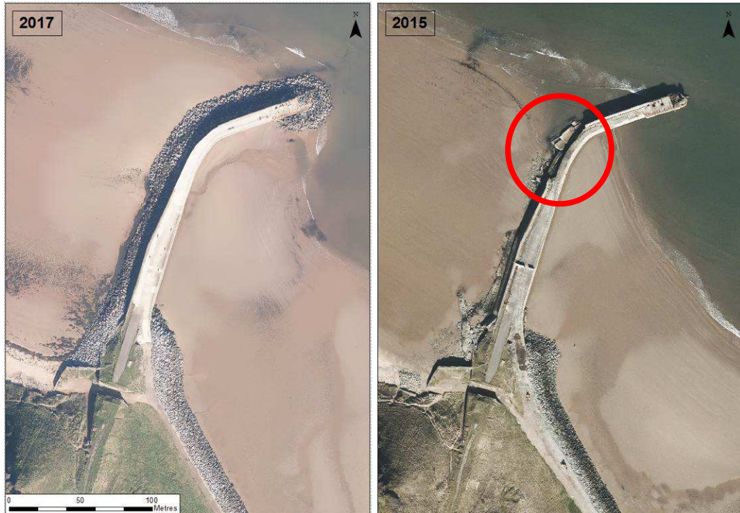
Figure 2-11 – Rock armourstone and concrete repairs at Skinningrove Jetty
