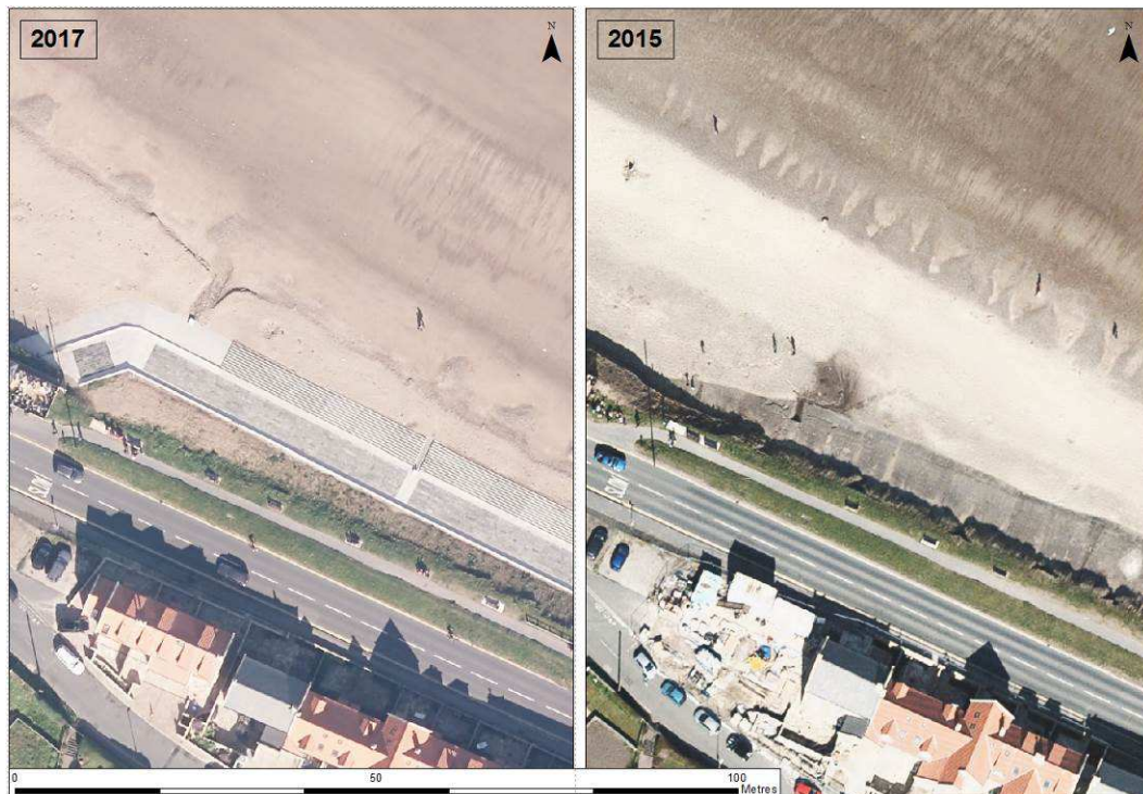
Figure 2-16 – Concrete revetment constructed at Sandsend Road
