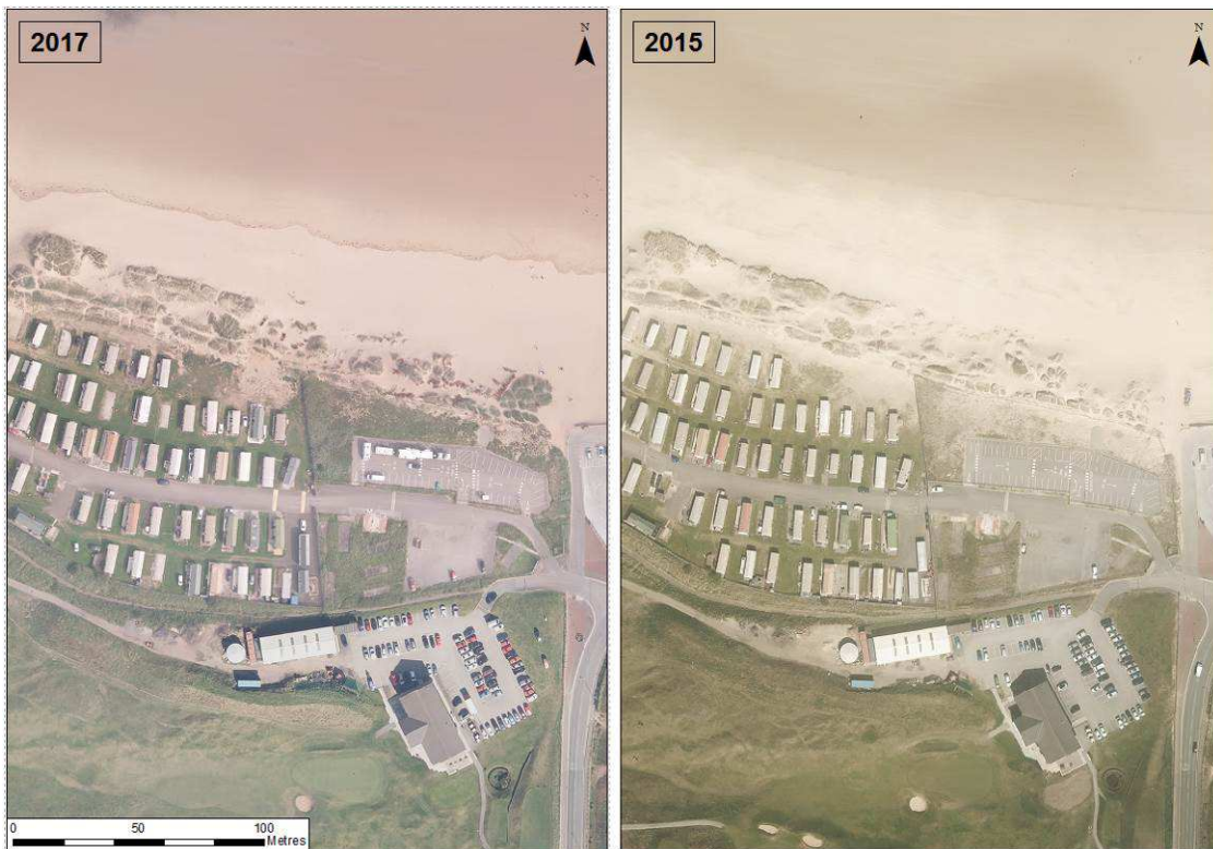
Figure 2-10 – Dune condition fronting eastern section of caravan park along Majuba section of Coatham Sands pre-dates January 2017 storms
