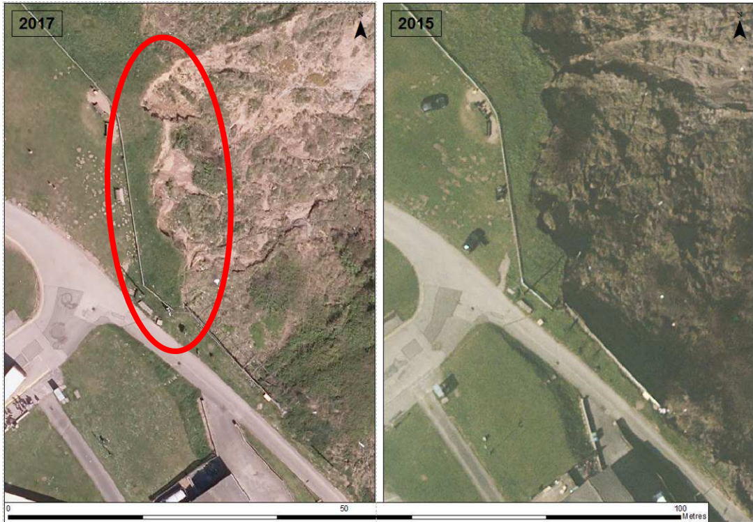
Figure 2-22 – Erosion at Flat Cliffs access road
