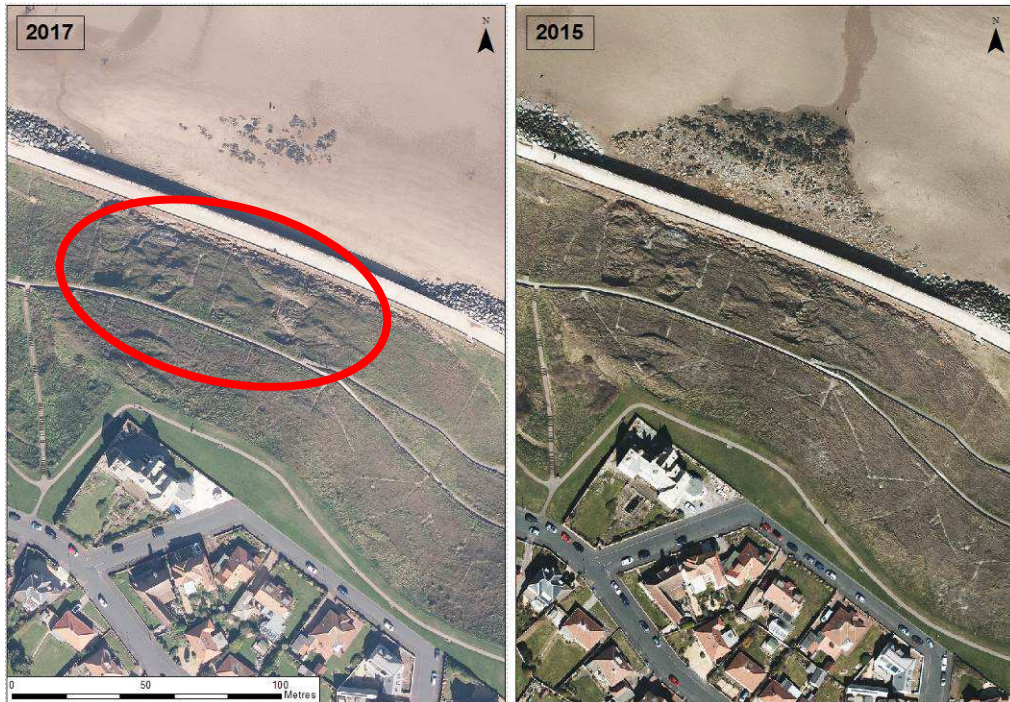
Figure 2-19 – Shallow slippages at the toe of Whitby West Cliff
