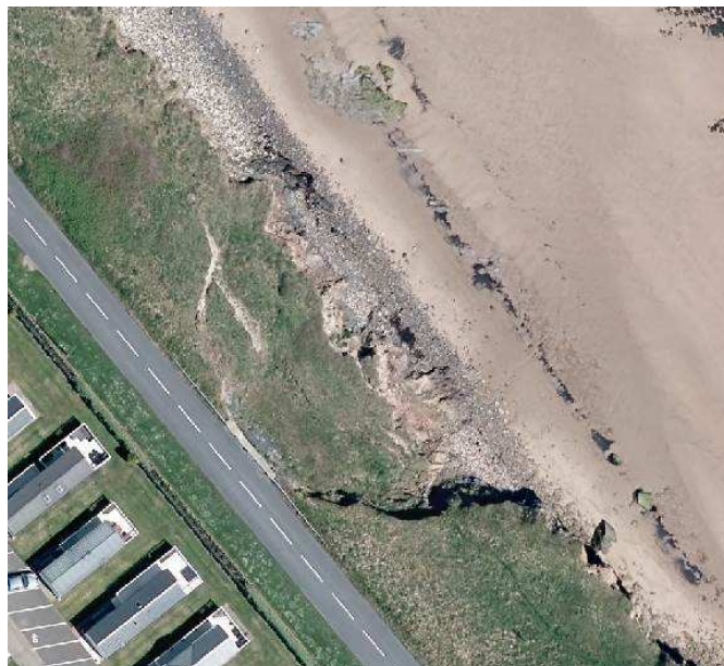
Figure 2-3 – Landslip at Cresswell impacting the road carriageway in 2017
